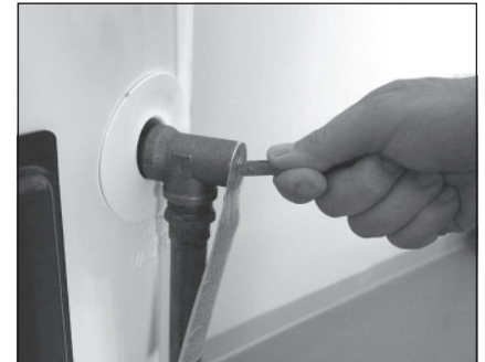
Figure 38 - T&P Relief Valve
